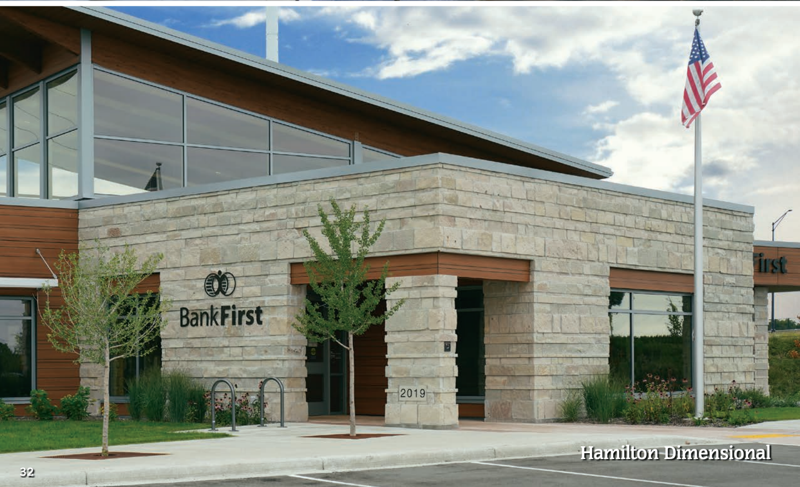
Fond du Lac Dimensional with Splits Hearthstone: Indiana Rockface
