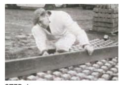
STEP 4 Level the paver grids on the sand bed. Keep them "pencil thickness" apart.
